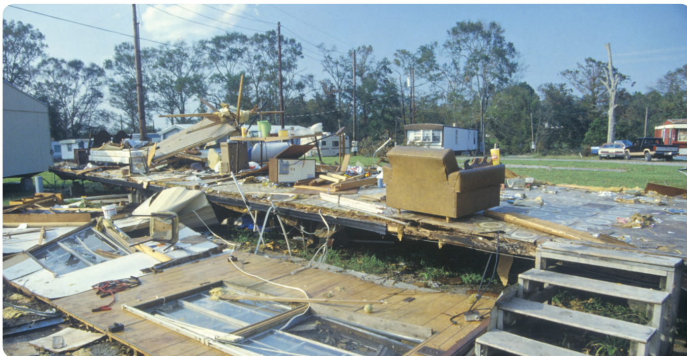
Hurricane Andrew left one trailer home in complete ruins and surrounding homes untouched in Jeanerette, Louisiana, USA in 1992. By Joseph Sohm / Copyright Shutterstock
