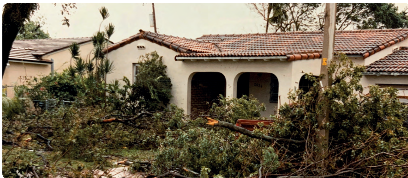
Extensive damage was caused by Hurricane Andrew in South Florida back in 1992. By wsbowles / Copyright Shutterstock
